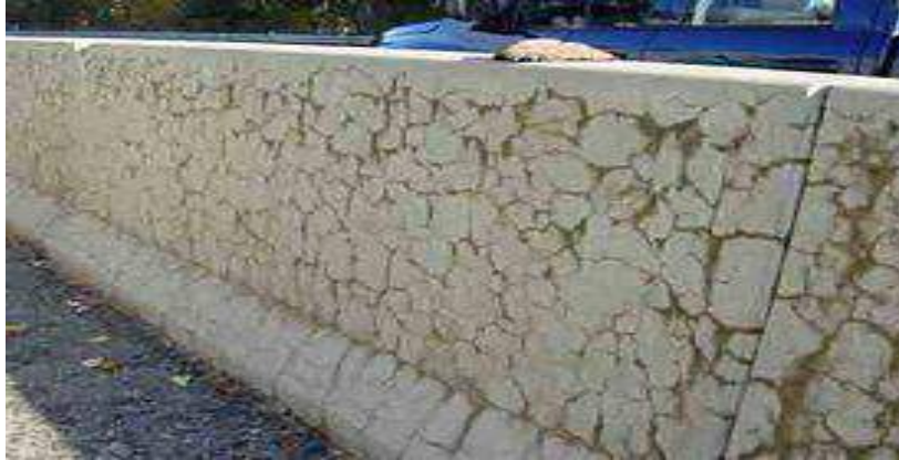
Typical effect of Alkali-Aggregate Reaction
